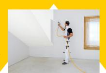
airless paint spraying system extracts materials directly out of the paint bucket or varnish container.
