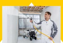
heavy, filled and high-viscosity materials such as bitumen and textured plaster over large areas.
